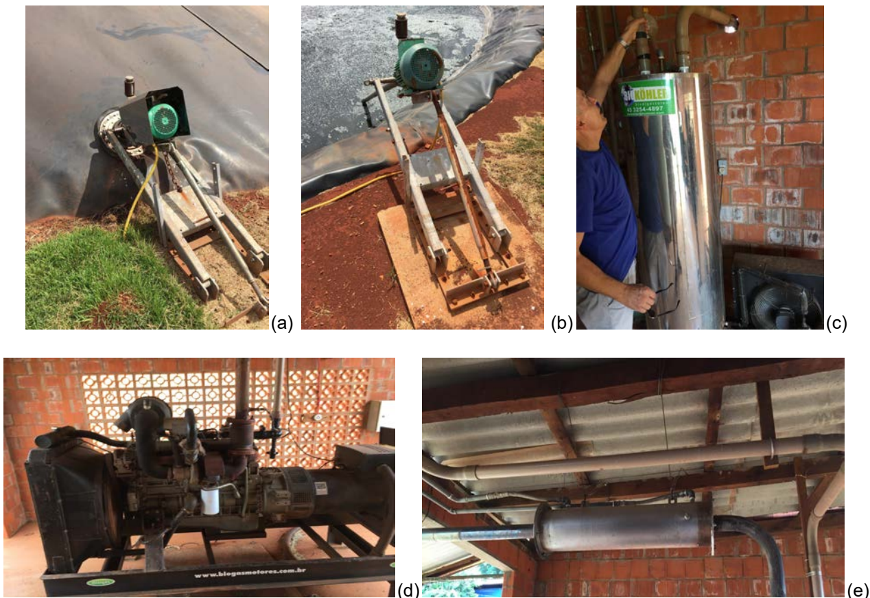
Figure 3.4.4 - Stein's Ceramics Biogas Plant Equipment (a) main digester SUMA mixer, (b) digestate lagoon SUMA mixer, (c) biogas desulfurization, (d) 75 kW generator (MWM engine + WEG magnetic generator) assembled by Biogas Motores and (e) heat exchanger (captures heat).
