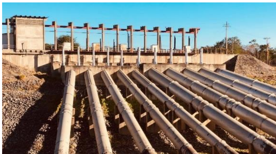
Water pump station Jaiba
