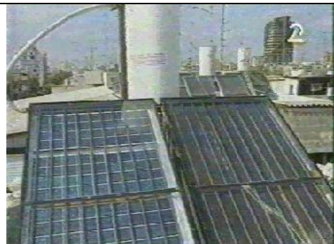
Figure 5: PVT collector from Millennium Electric, showing both air and water connections.
