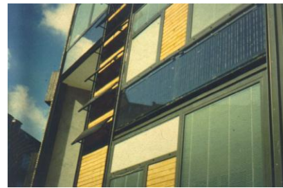
Principle for ventilated solar wall with integrated PV panel in The Yellow House Note that the PV Panel is placed on the inside of the air gap
