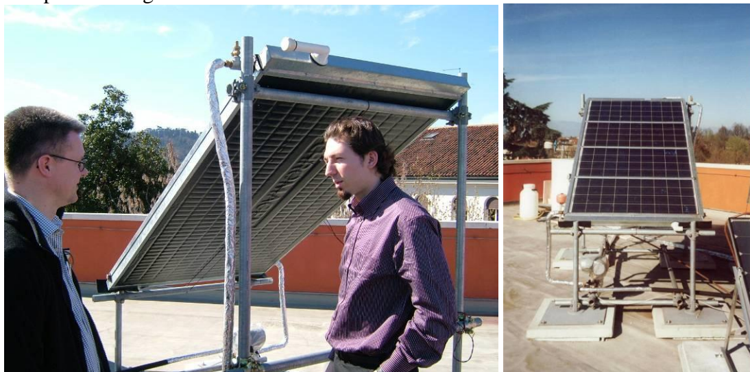
Figure 5: PVT collector from Millennium Electric, showing both air and water connections.
