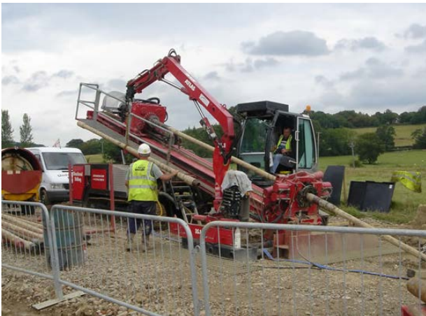
Figure 11 HDD tools and machinery
