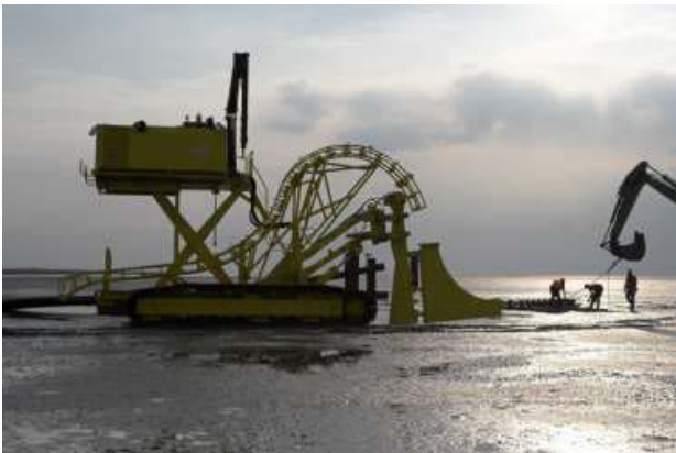
Figure 33 Vibration plough on tracks
