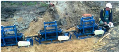
Figure 16 Typical cable tensioners
