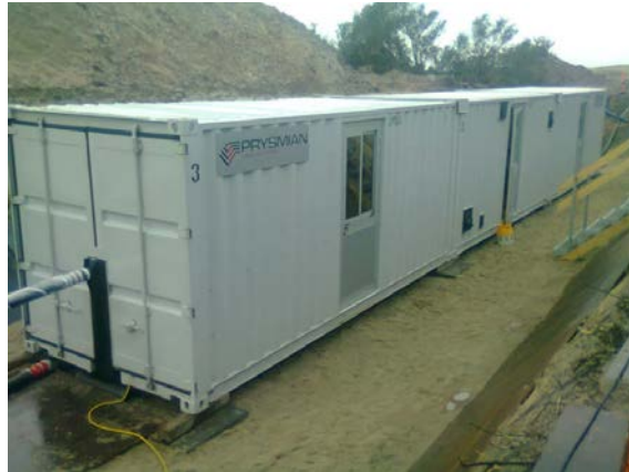
Figure 21 Typical jointing containers
