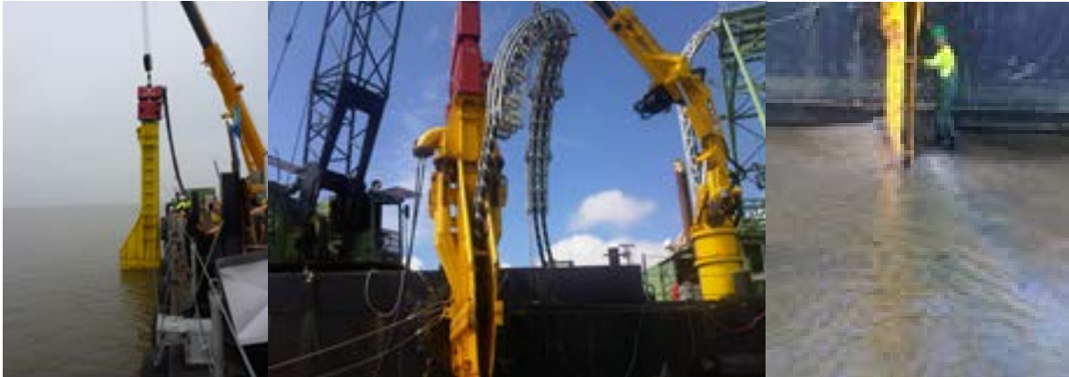
Figure 32 Vibration plough deployed from a barge
