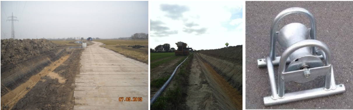
Figure 15 Pull in wire and rollers (left), backfilling before cable pull in (middle), typical roller (right)
