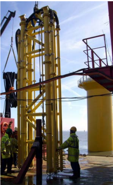
Figure 38 Air lift
