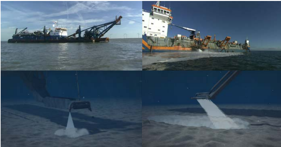
Figure 37 Mass flow excavation by a converted Suction Dredger or Hopper Dredger
