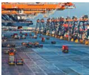
Source: Europe Container Terminals BV, Rotterdam
