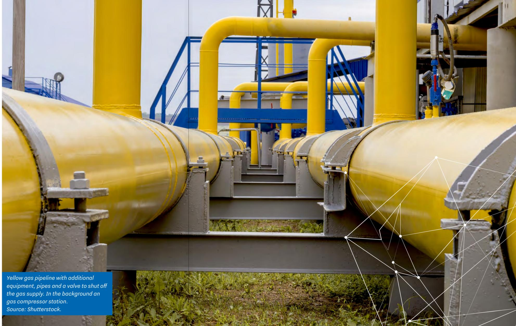
Yellow gas pipeline with additional equipment, pipes and a valve to shut off the gas supply. In the background an gas compressor station. Source: Shutterstock.
