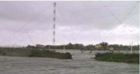
Dike failure in 2004 TP Mindull
