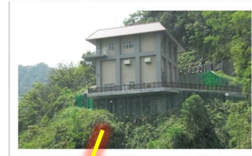
Stratified water intake shaft
