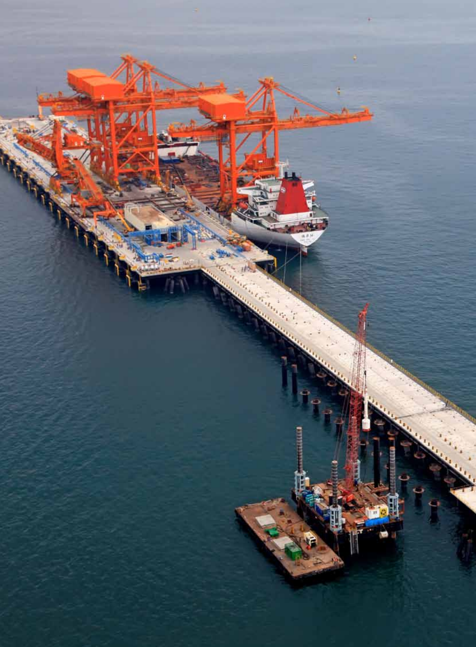
Soha iron ore jetty, Royal Haskoning (Directorate General of Ports, Ministry of Transport and Communications, Sultanate of Oman)
