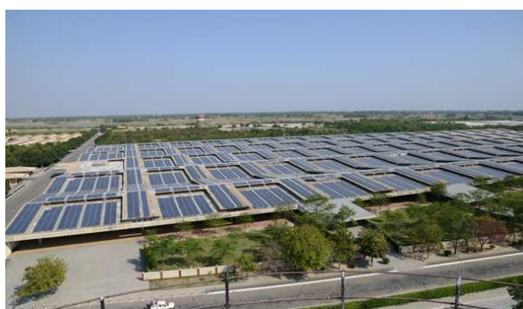
Figure 1 – 7.5 MW rooftop system (Beas, Punjab)
