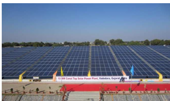
Figure 2 – 10 MW canal-covering system (Vadodara, Gujarat)
