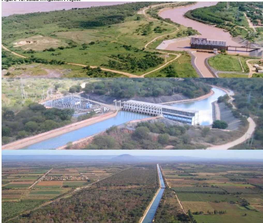
Figure 13. Jaiba Irrigation Project
