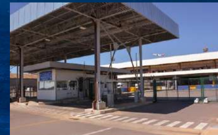
Access gate with security control
