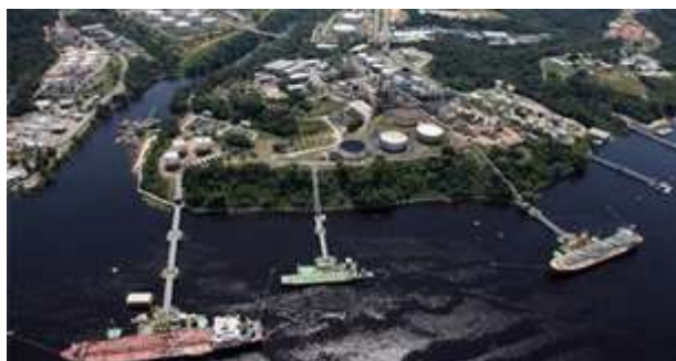
Source: REMAN – Refinaria Isaac Sabbá, Petrobras, 2020.
