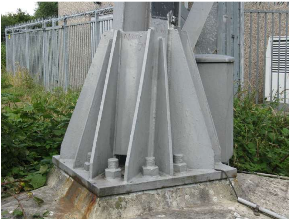
Figuur 2 Picture of foot detail tower 49 (similar to tower 12 and 13)
