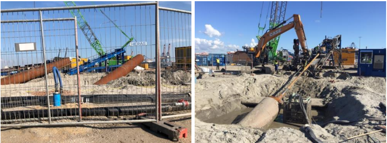
Figure 25 - Examples of reamer in HDDs
