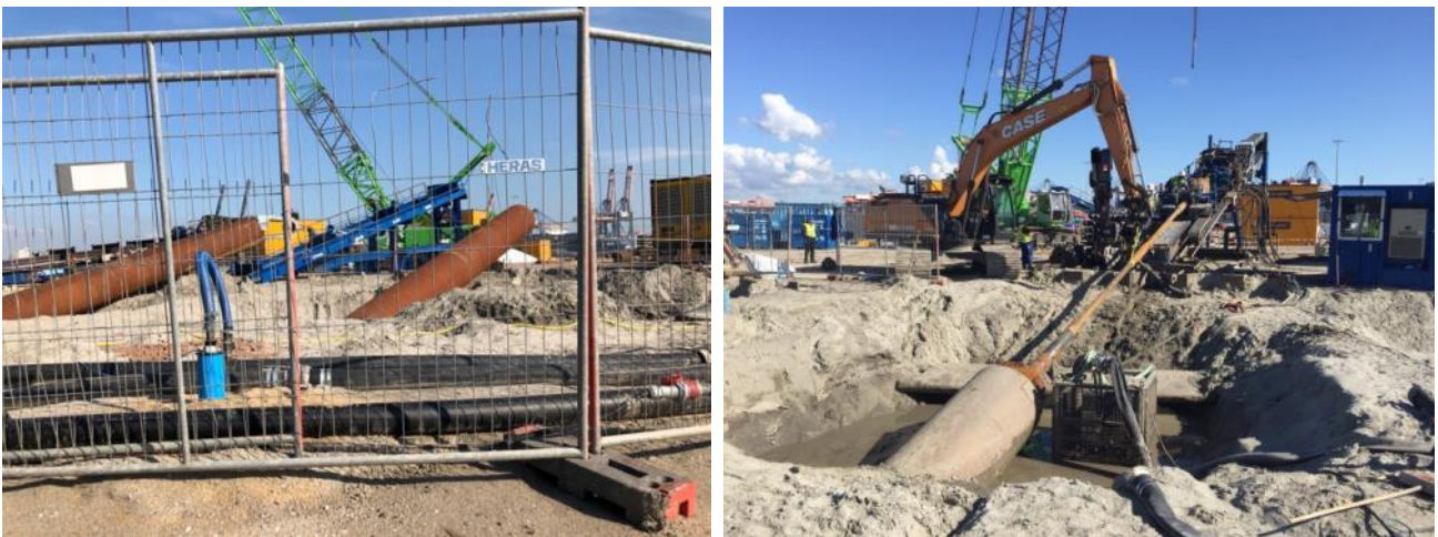
Figure 25 - Examples of reamer in HDDs
