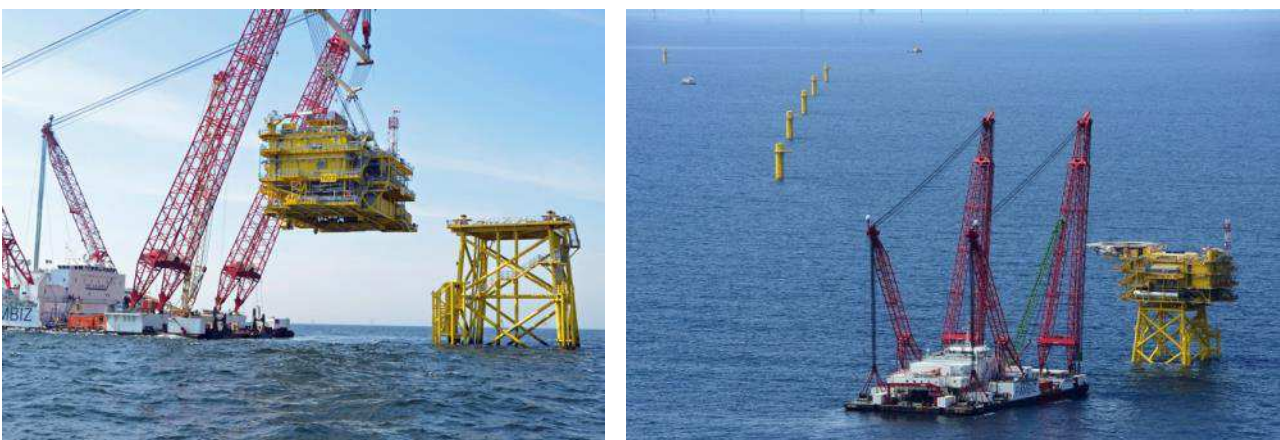
Figure 60 Installation of topside
