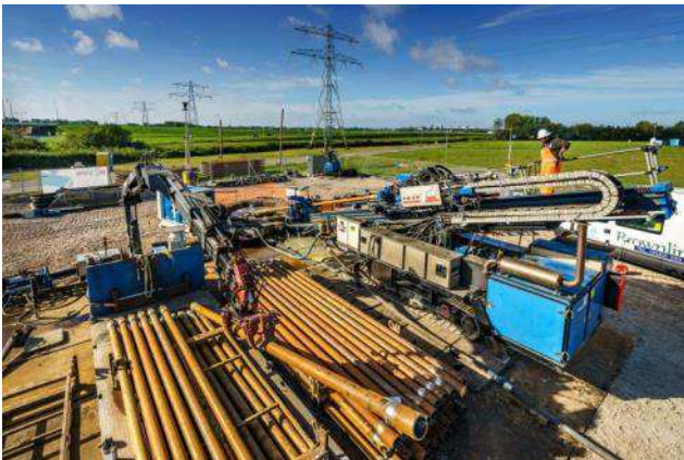
Figure 26 Example of HDD entry and exit point
