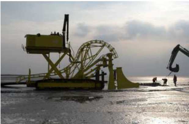
Figure 51 Vibration plough on tracks
