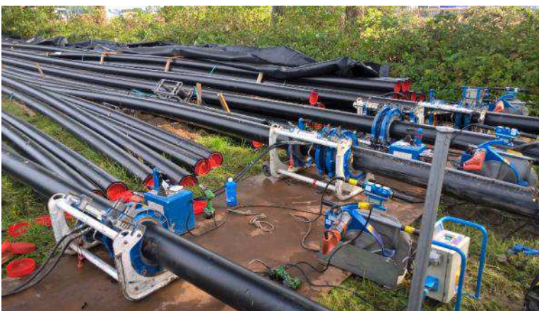
Figure 27 Welding of HDPE ducts
