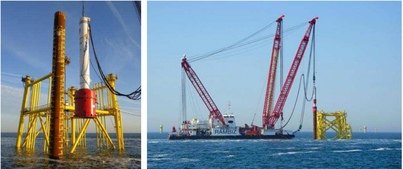
Figure 59 Piling of jacket
