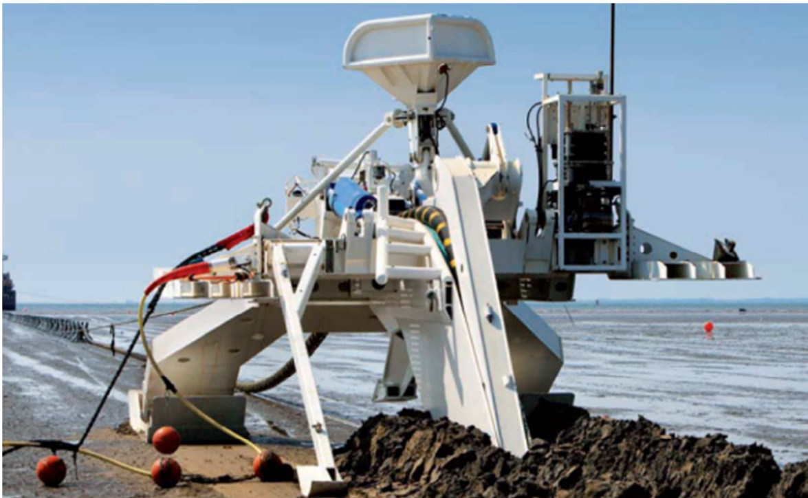
Figure 42 Sea Stallion cable plough
