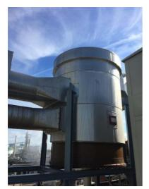
Exhaust gas flow Exhaust gas inlet temperature Exhaust gas outlet temperature Air inlet temperature Air outlet temperature Duty Energy savings (@ 0.50 €/m<sup>3</sup>) Avoided yearly CO<sub>2</sub> emission 13,200 kg/hr 59 °C 56 °C 10 °C 56 °C 169 kW 69,200 €/yr 267 ton/yr
