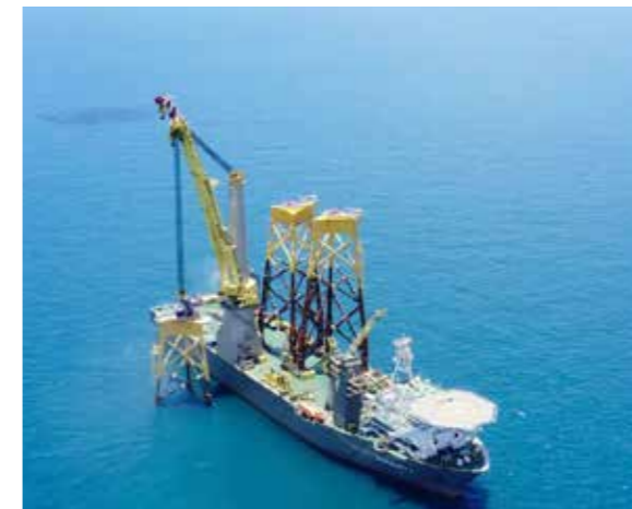
Bokalift 2 installing jacket foundations at Changfang and Xidao. Source: Boskalis
