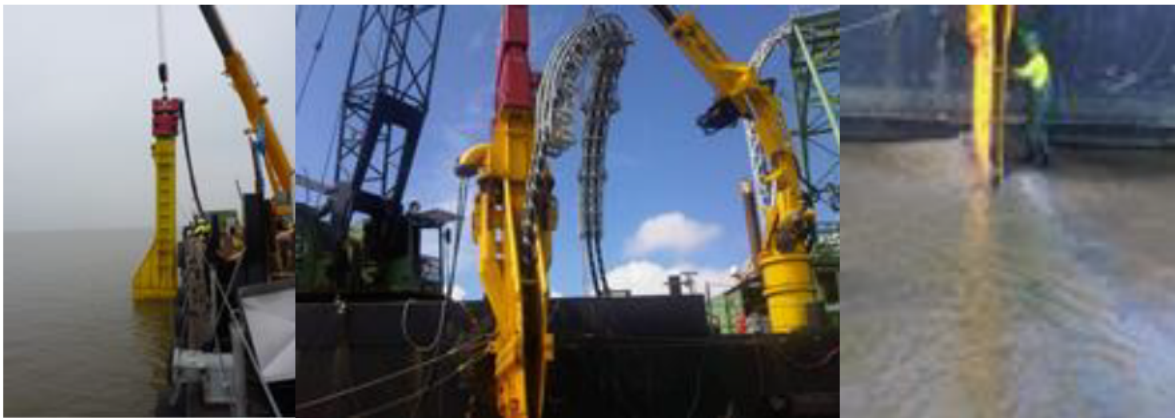
Figure 53 Vibration plough deployed from a barge
