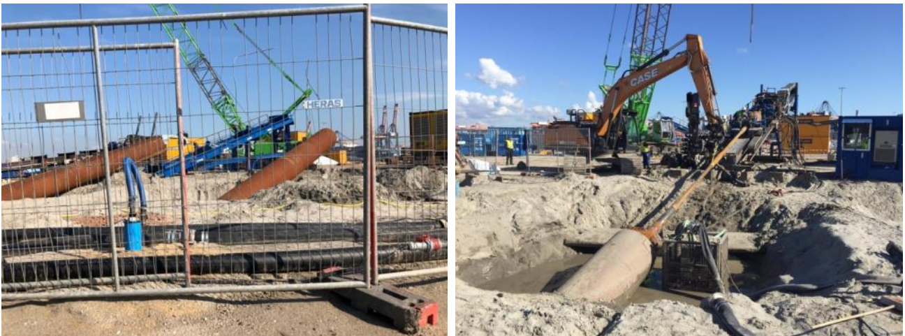
Figure 25 - Examples of reamer in HDDs
