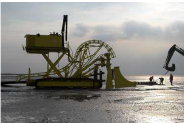
Figure 54 Vibration plough on tracks
