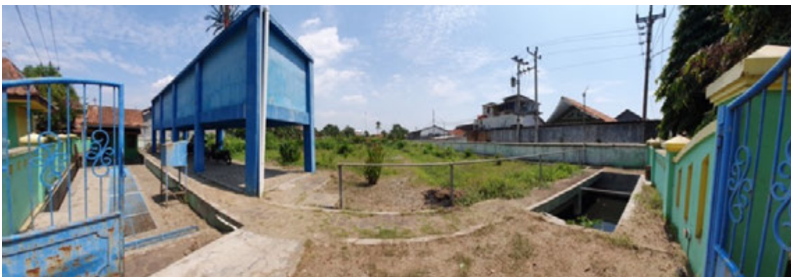
Figure 24 Constructed wetlands in WWTP Jenggol
