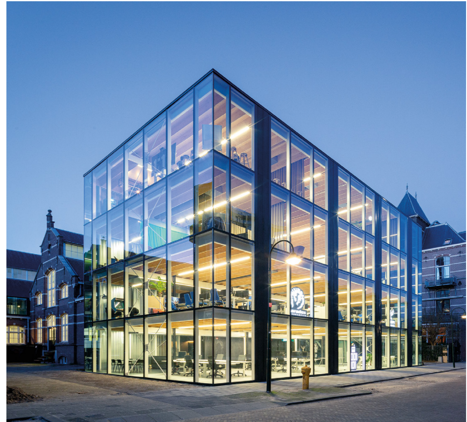
Photo: Bouwdeel D, a fully demountable office building in Delft, constructed entirely from a prefabricated steel structure and prefabricated laminated wooden floors of Laminated Veneer Lumber (LVL) elements. Credits: cepezd
