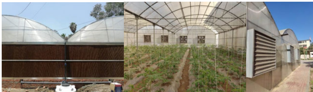
Figure 25 Cooling systems (pad and fans) ©Delphy
