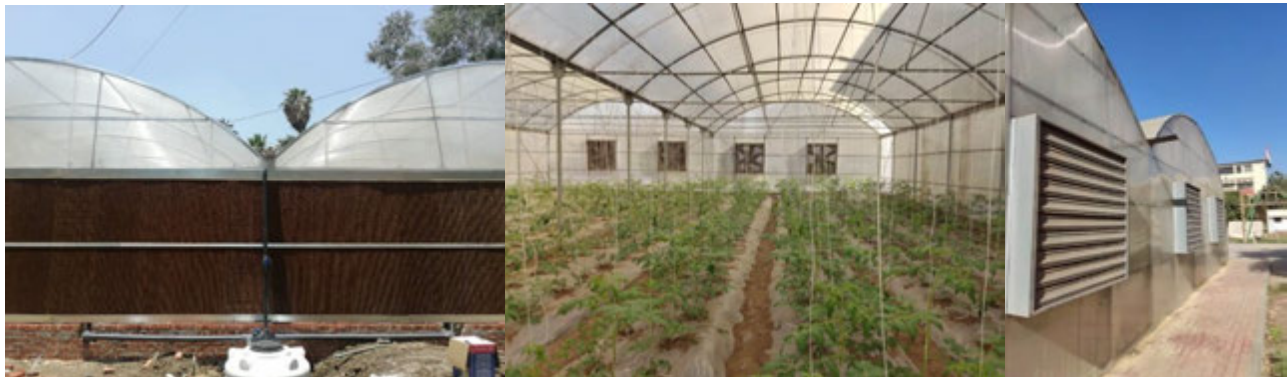
Figure 25 Cooling systems (pad and fans) ©Delphy
