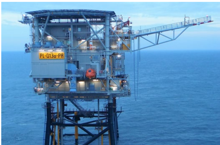
An existing oil and gas platform off the Dutch coast is being converted to the world's first offshore hydrogen platform. Electricity generated by offshore wind turbines will be used to convert seawater into demineralised water and to power a 1-MW electrolyser producing clean hydrogen.
