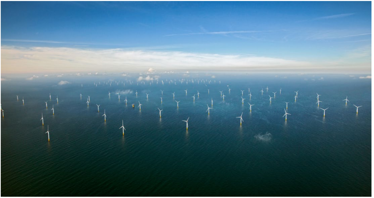
The offshore wind area "Ten noorden van de Waddeneilanden", located 56 km off the coast of the north of the Netherlands, has been designated for large-scale offshore hydrogen production. The preferred location could provide up to 500 MW of electrolysis capacity to be operational in 2031. The sheer size would make it world's largest offshore hydrogen production location. (Photo: Gemini Windpark)
