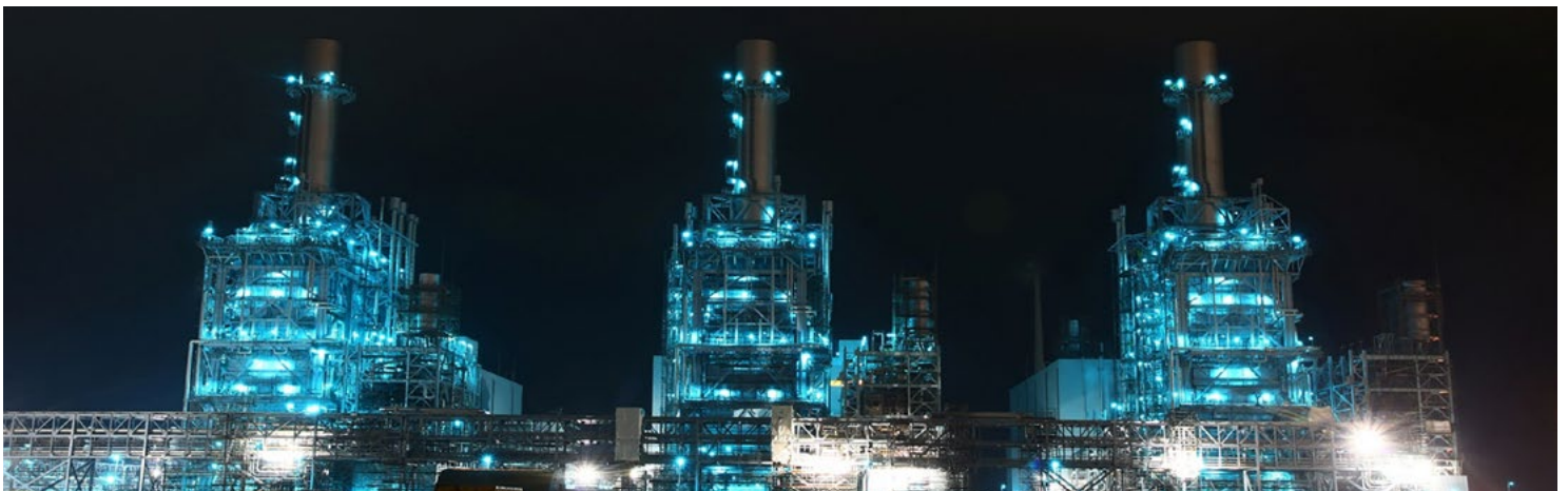
In the Eemshaven, the port in the north of the Netherlands an existing gas-fired power plant is being prepared to convert to hydrogen. After acquiring the plant from Vattenfall in 2022, RWE continues to pursue the ambition of having the first of the plant's three 440-MW units run on (low-carbon) hydrogen. By converting the remaining units and switching to clean hydrogen by 2030, this is likely to become the world's first carbon-neutral hydrogen-fuelled power plant.
