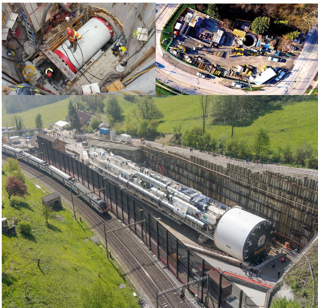
Figuur 2-11 Van 54-inch Herrenknecht AVN slurry microtunnel machine ( https://tunnelingonline.com/microtunneling-on-a-curve/ ) tot 20 m tunnelmachine ( https://amberggroup.com/news-events )
