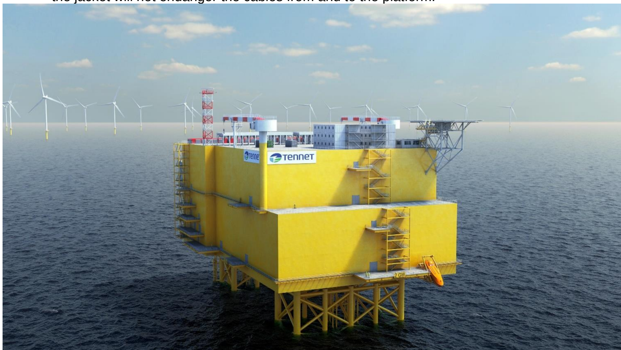
Figure 4 Artist impression of 2 GW HVDC offshore platform concept
