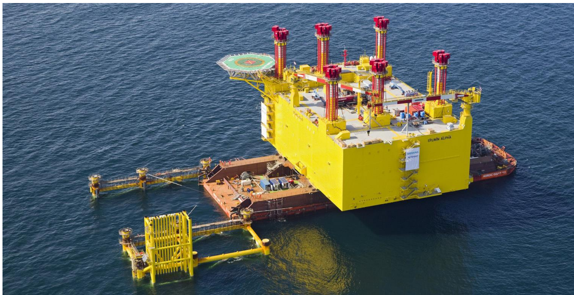
Figure 13 - Floatover installation with barge of the Sylwin Alpha topside
