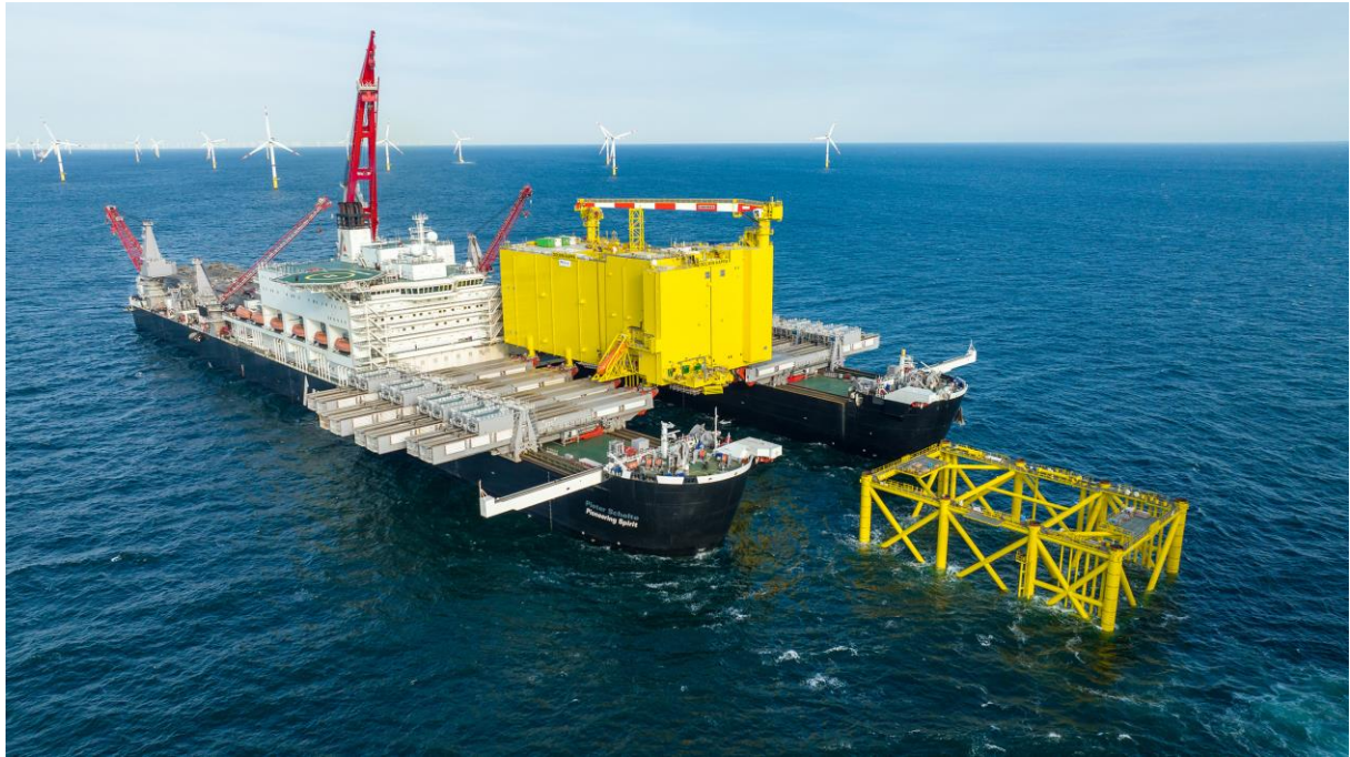
Figure 14 Catamaran installation with the Pioneering Spirit
