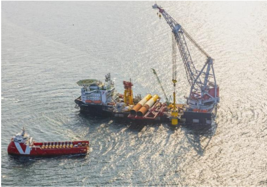
Figure 10 - noise mitigation vessel operating during pile driving
