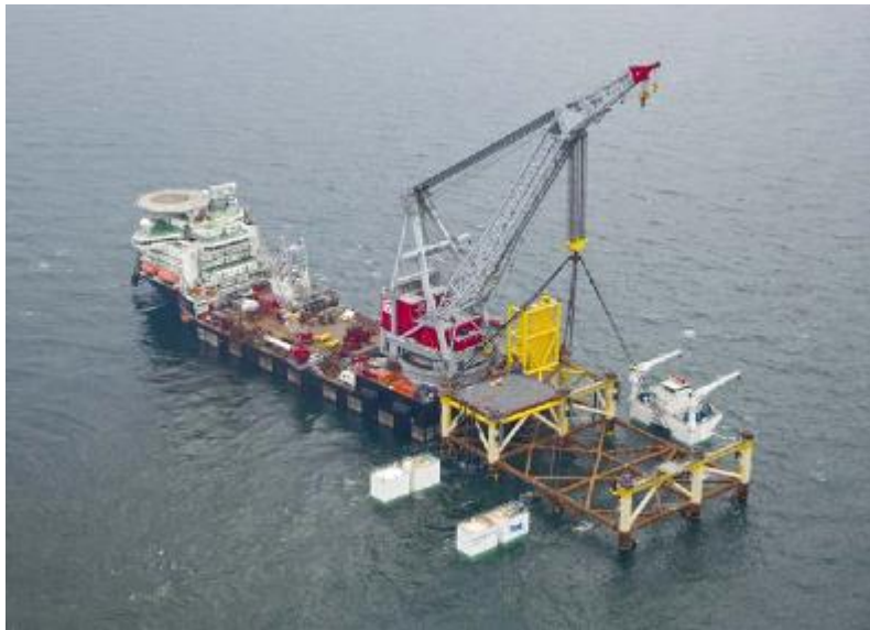
Figure 8 Installation of floatover jacket by heavy lift vessel (Sylwin Alpha Platform 900MW)
