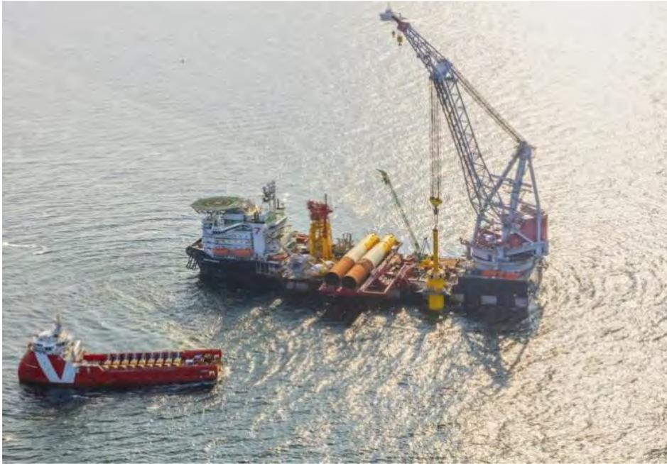
**Figure 10 - noise mitigation vessel operating during pile driving**
