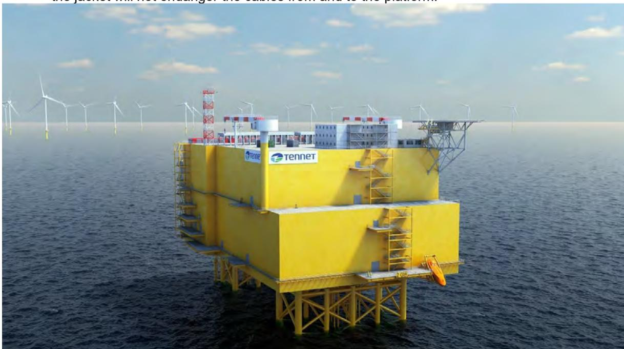
Figure 4 Artist impression of 2 GW HVDC offshore platform concept
