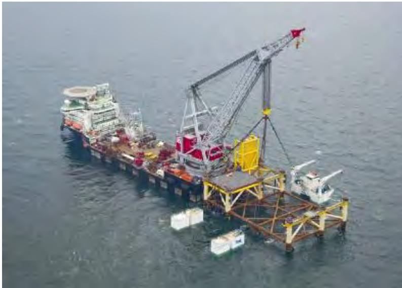
**Figure 8 Installation of floatover jacket by heavy lift vessel (Sylwin Alpha Platform 900MW)**
