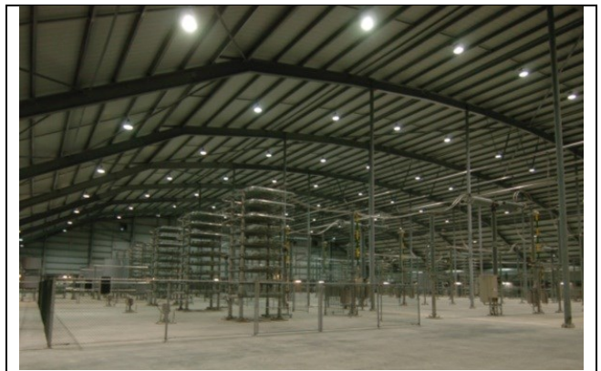
Afb. 2.29: Condensatoren in de Filterhal
