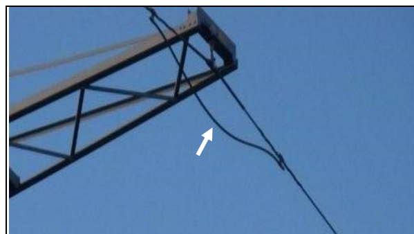
Afb. 3.23: Bretelle-trillingdemper
