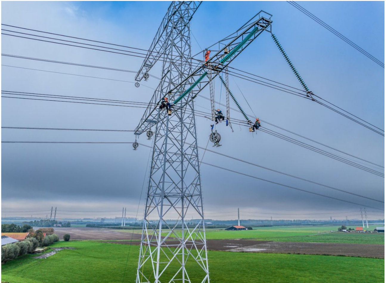
Figuur 5.4: Ophangen isolatoren of isolatorkettingen
