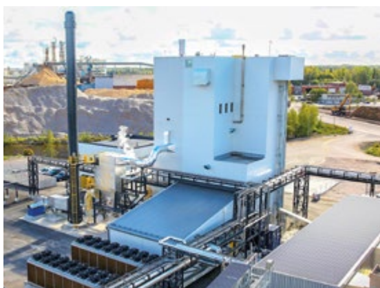
BTG Bioliquids' fast pyrolysis technology can convert different types of residues into a homogeneous, standardised bio-oil for heat, power, and refinery co-processing. Its reference plant in the Netherlands has already produced thousands of tonnes of oil, while the technology has also been deployed in Scandinavia and Malaysia. Parent company BTG, meanwhile, has supported biomass projects in over 80 countries as consultant and project developer.
