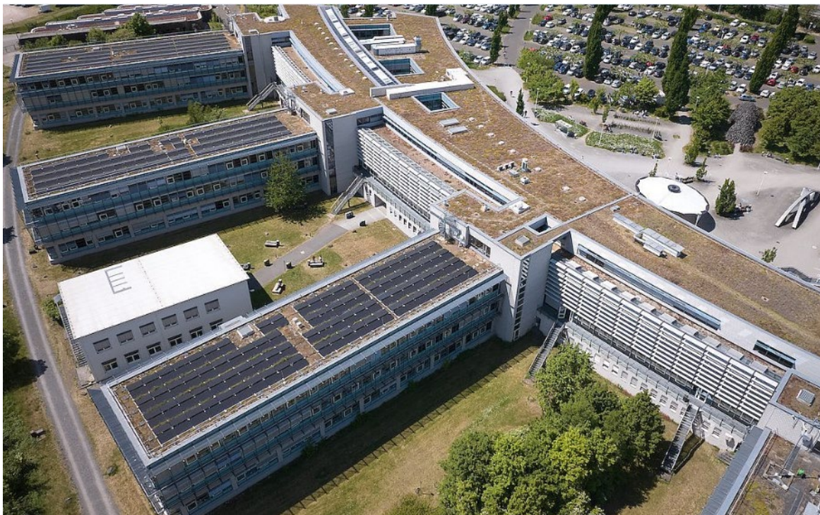
Figure 10: Photovoltaic panels installed on the rooftops of the Koblenz University of Applied Sciences 106
