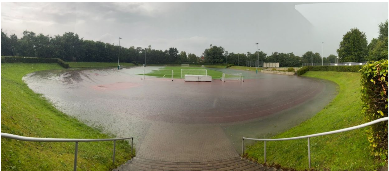
Figure 13: Hein-Klink Stadium was designed to serve as emergency overflow for rainwater drainage 129
