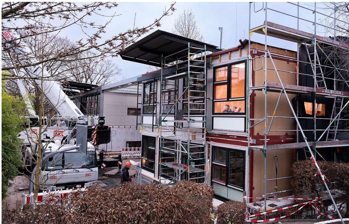
Figure 12: Serial refurbishment of a daycare centre in Frankfurt am Main 125
