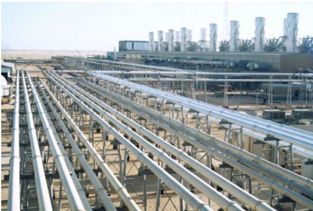
Figure 20: Example of several parallel GIL circuits (GE)
