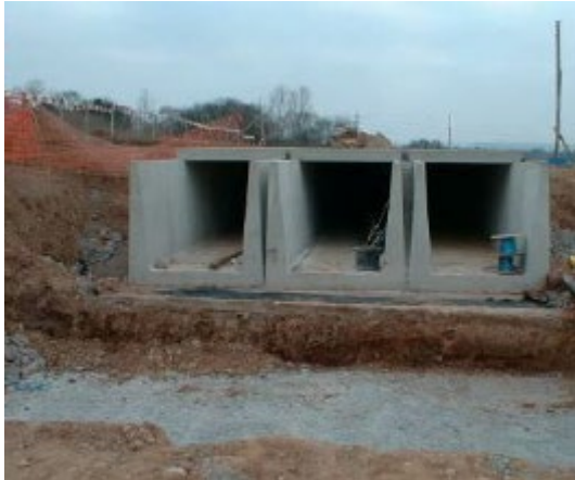
Figure 19: Example of concrete duct under construction for GIL installation (GE)
