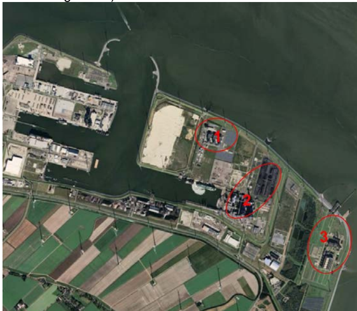
Figure 5.1 Overview existing plants in the project area.
