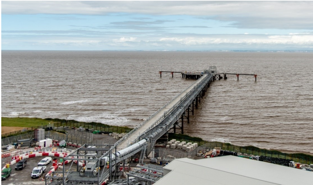
Figure 10: Temporary jetty (HPC) 15
