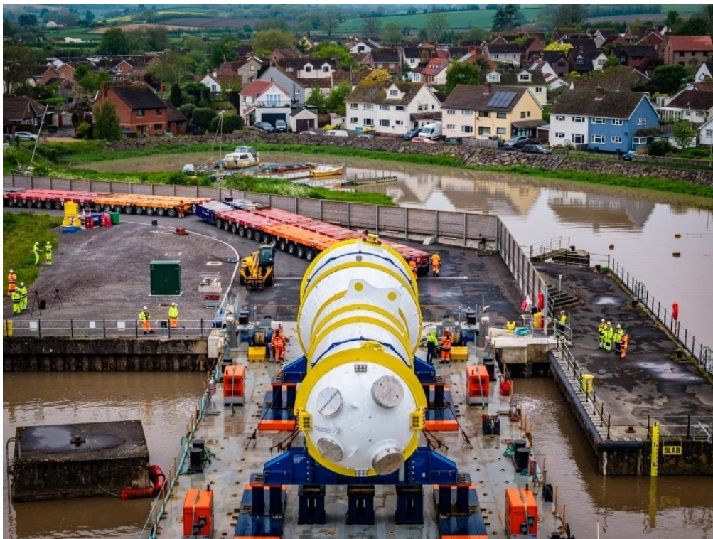
Figure 11: Steam generator delivered by barge to Combwich Wharf (HPC) 15
