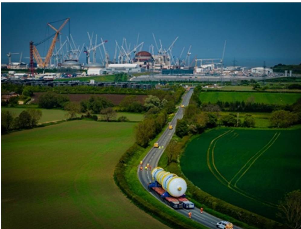
Figure 9: Steam generator delivered to HPC construction site 15
