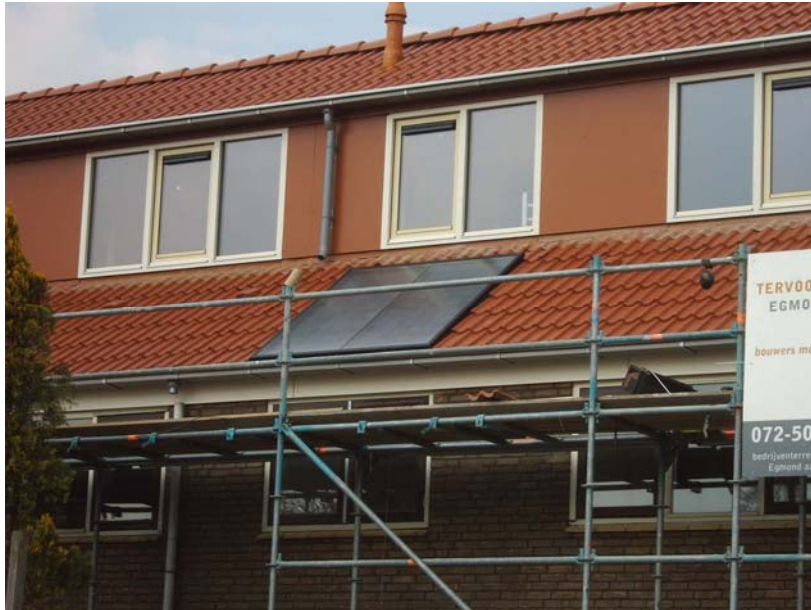
Figure 109: Final result of the PVT installation
