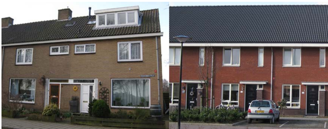
Figure 24: Traditional building style for retrofit (left) and new construction (right)
