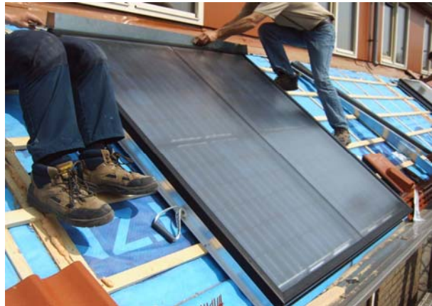
Figure 103: Positioning of PVT panel
