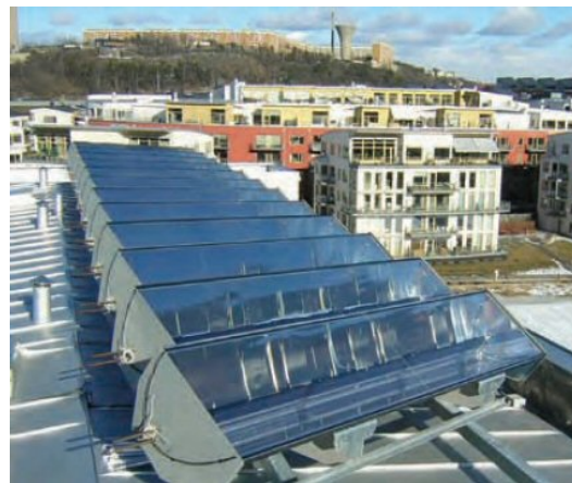
Figure 14: Ventilated PV with heat recovery [ 16] Figure 15: PVT concentrators [ 2]
