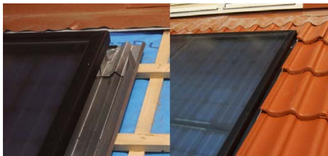
Figure 23: PVT flashing set
