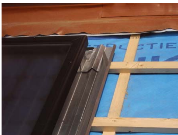
Figure 104: Top and side gutter
