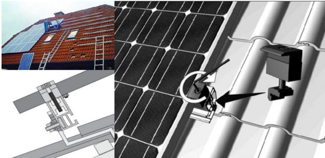
Figure 19: On roof installation – VarioSole system [ 37]
