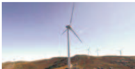
© EDF Energies Nouvelles – AltoMinho Windpark
